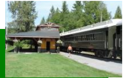
Metaline Falls Train Depot Metaline Falls, WA 99153
